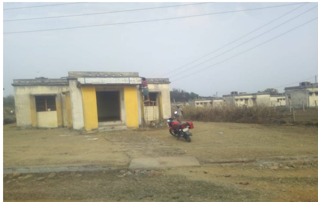
Resettlement House under repairing at Parang
