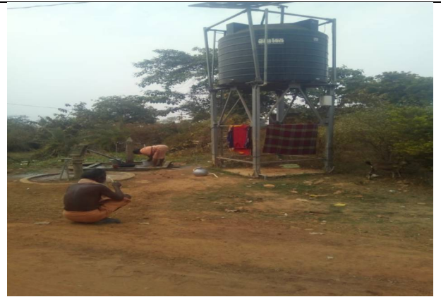
Water Facility in Dhobamalia
